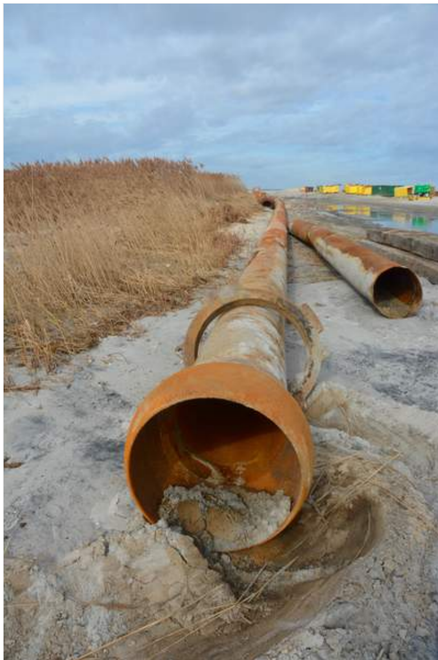
Pipes used for dredging are piled up and ready for use. (Photo by: Ron MacArthur)
