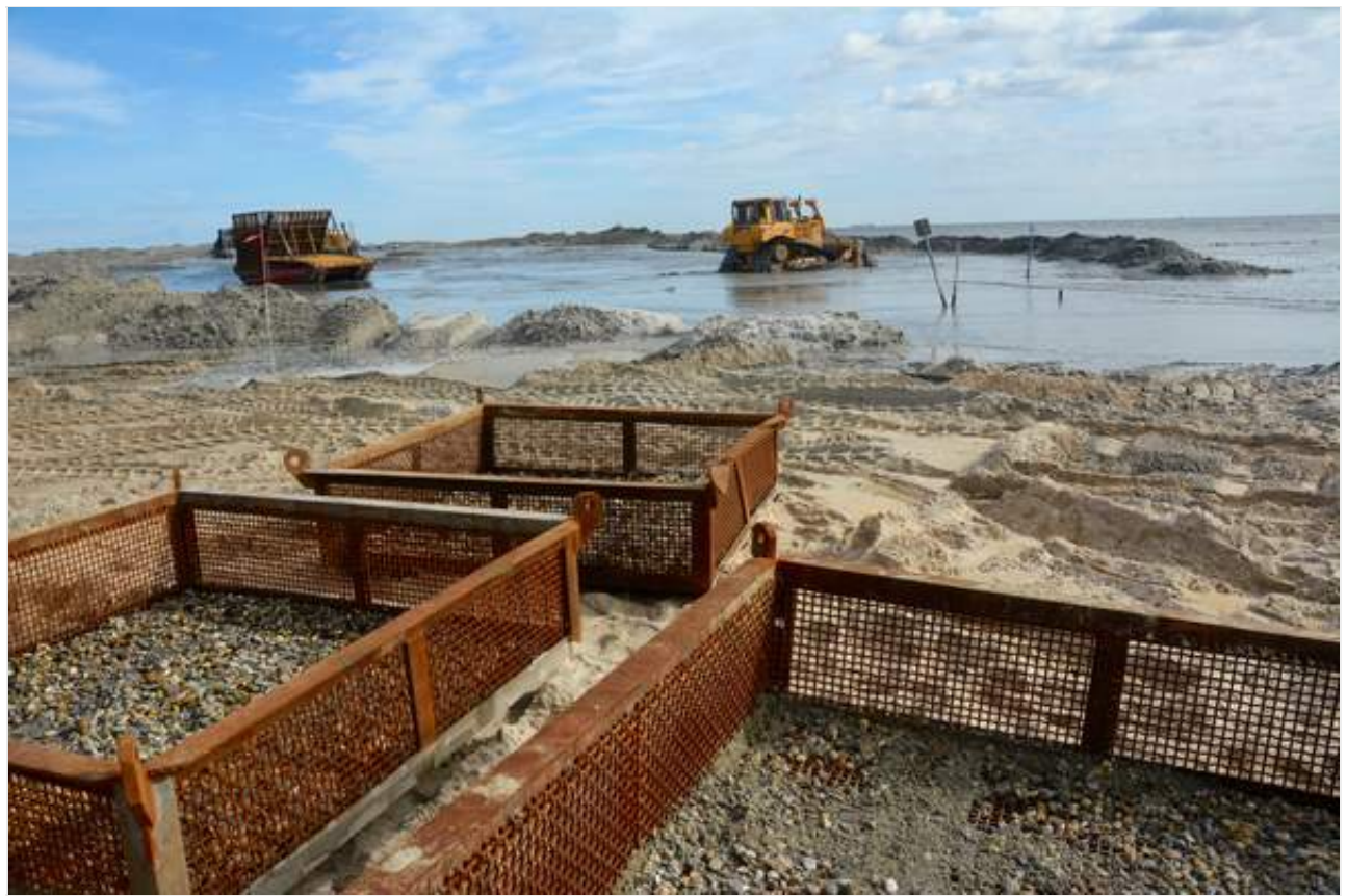
Large stones are filtered out of the sand before it is used on the beach. ( Photo by: Ron MacArthur )
